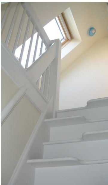
Special alternating tread stair minimizes loss of landing space
